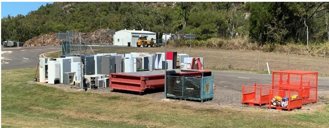
Figure 17: Waste separation area transfer station. White goods, air conditioners, tyres, electronics and gas canisters are separated.
